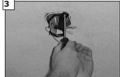
Use metal outlet box suitable for fan support (must support 35 lbs). Before attaching fan to outlet box, ensure the outlet box is securley fastened by at least two points to a structural ceiling member (a loose box will cause the fan to wabble). Use only the screws provided with the outlet box.
